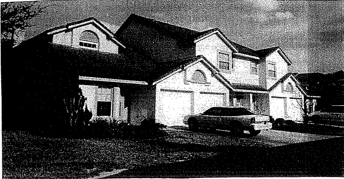
Similar Construction but with Regular Shingles in lieu of a Tile Roof
