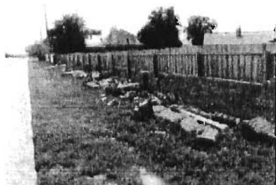
Photo No. 2: Partially collapsed section of wall.
