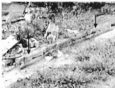
Photo No. 4: Arrows highlight full bedding of mortar bonded to bottom course of masonry failure.
